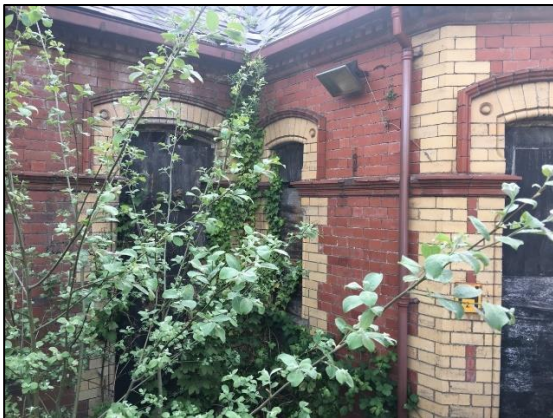
Photo 15 Open window on eastern elevation
