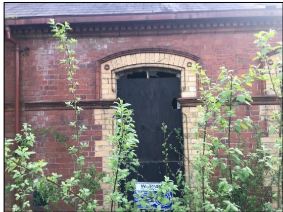
Photo 14 Open window on eastern elevation
