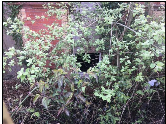
Photo 16 Open window on eastern elevation
