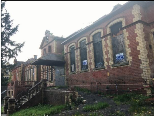
Photo 1 Front (south-eastern) elevation
